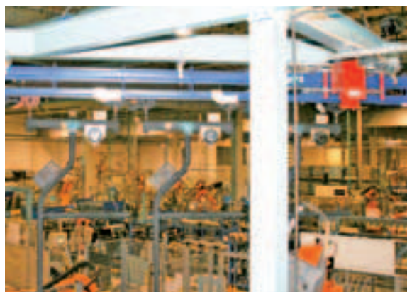
Thanks to the Turck RFID system, Tower Automotive was not only able to increase production at the same cost, but also make it more reliable
